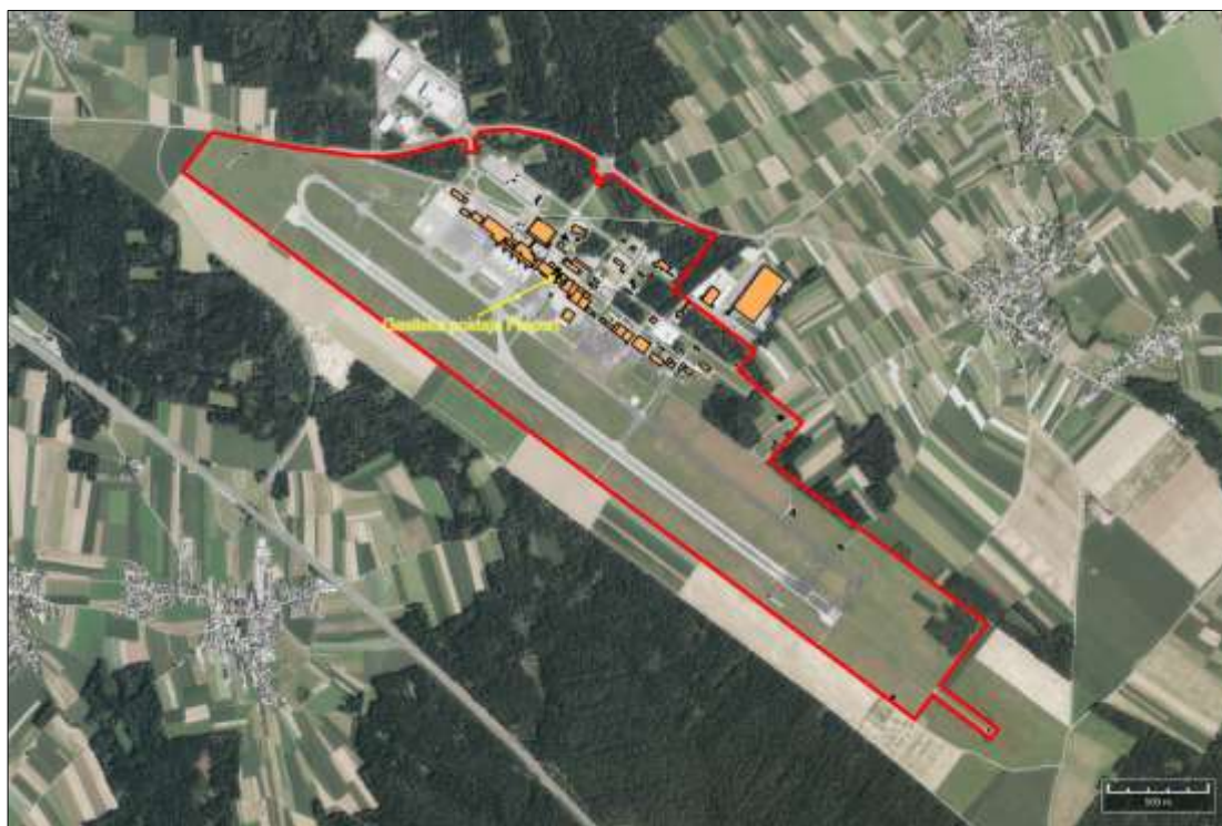
Picture 3: The area of operation of Airport Rescue & Fire Fighting of Fraport Slovenija
